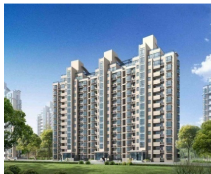
Building water supply
